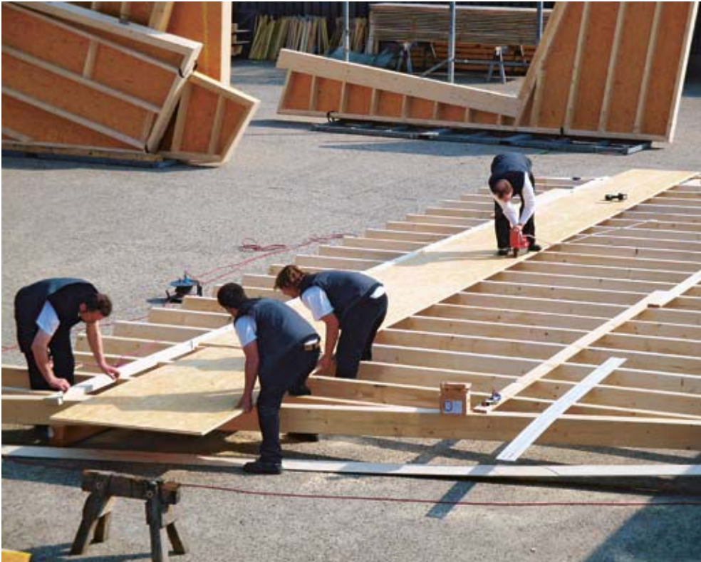
Wood frame construction – prefabrication and assembly
