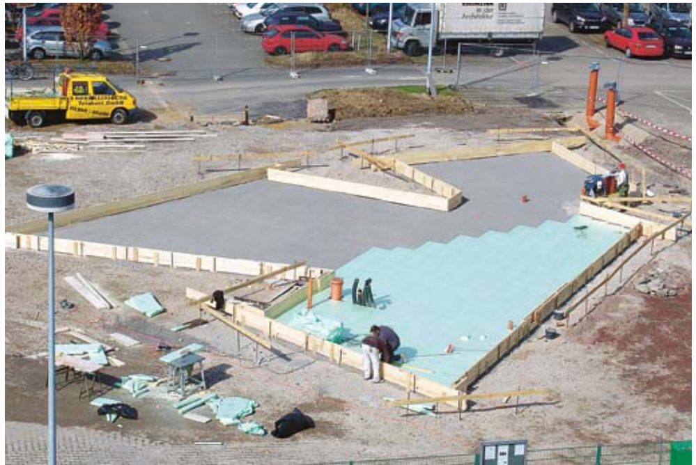
Work on the ground slab in progress
