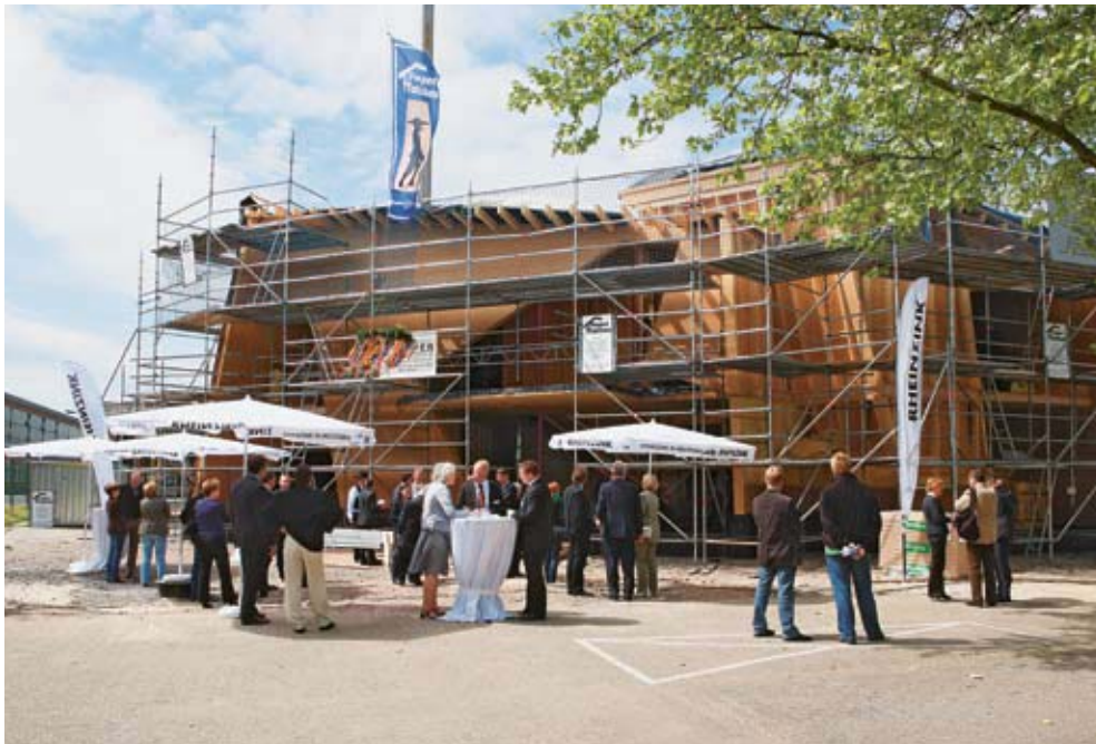
A workman's tradition – the last nail is hammered in
