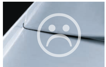
Gable roof ridge without expansion area and insufficient installation height
