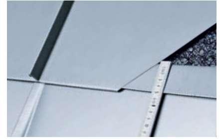
Cross joint designed as a single seam
