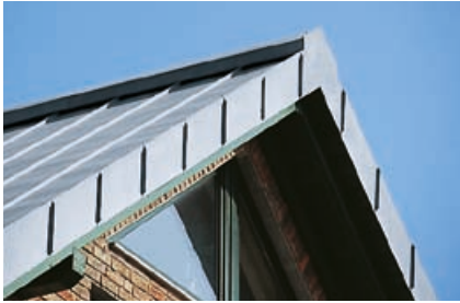
Ridge for a vented gable roof – high design with ventilation cross-sections
