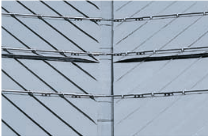
Valley gutter recessed on structured mat
