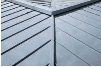
Hip with batten and coping profile
