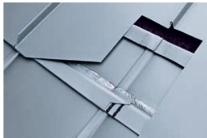
Detail optimization: soldered continuous cleats
