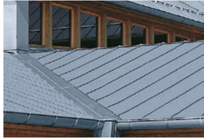
Valley with a single seam and soldered continuous cleat
