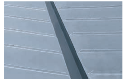
Valley gutter with lined overflow gutter
