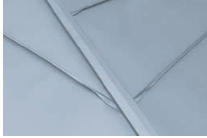
Hip without batten, with coping profile
