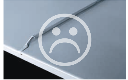
Gable roof ridge – eaves termination
